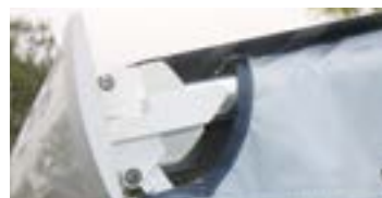
Optimal awning connection
